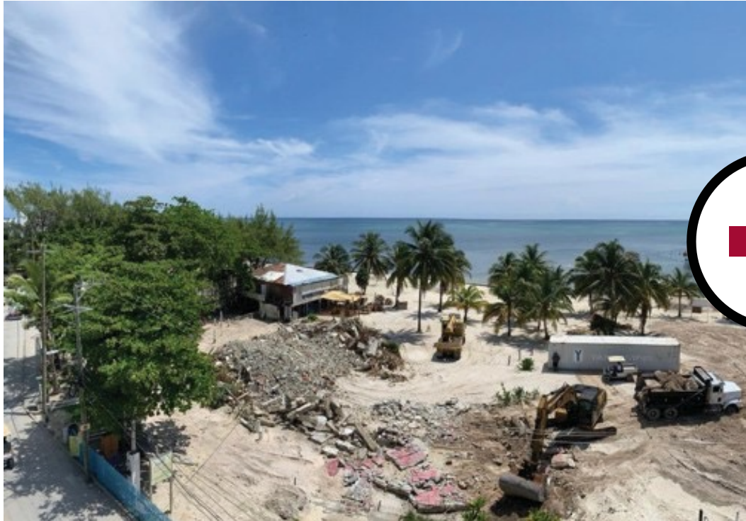
TEAR DOWN AND SITE PREP
